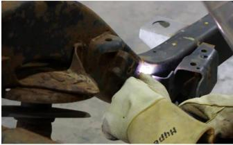
Begin cutting away the upper control arm mount bracket as close to the frame rails as possible.
