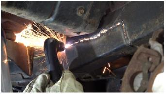
You will need to cut a small gap at the back of the body mount bracket and engine mount bracket to slide your new leaf spring mount section behind the brackets for welding.
