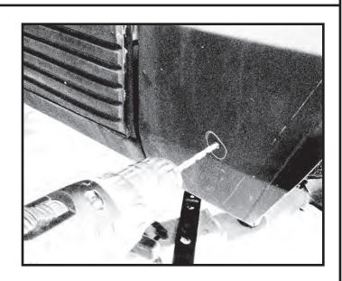
Step 23. Drill the mounting holes using a 3/16" drill bit.
