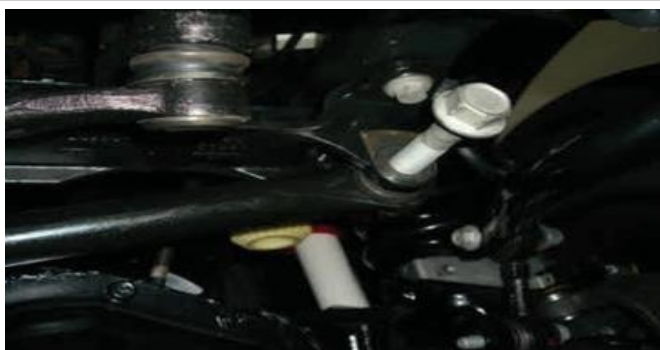
Loosen track bar at the frame.
