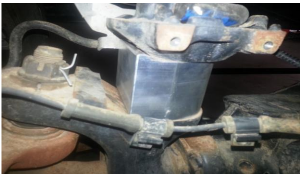
Place billet spacer on axle under spring perch. Secure with the provided hardware and torque to spec. Re-install the front spring and raise axle to hold in position.
