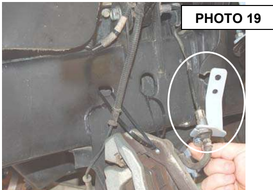
Install the line on the new bracket.
