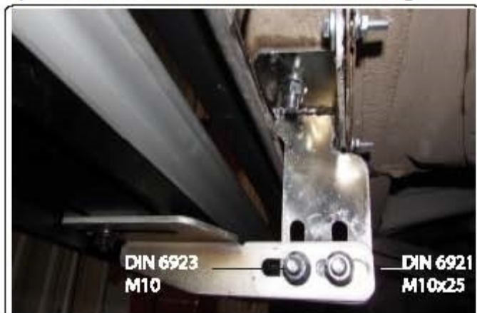
7) Attach lower portion with M10 hardware do not tighten yet
