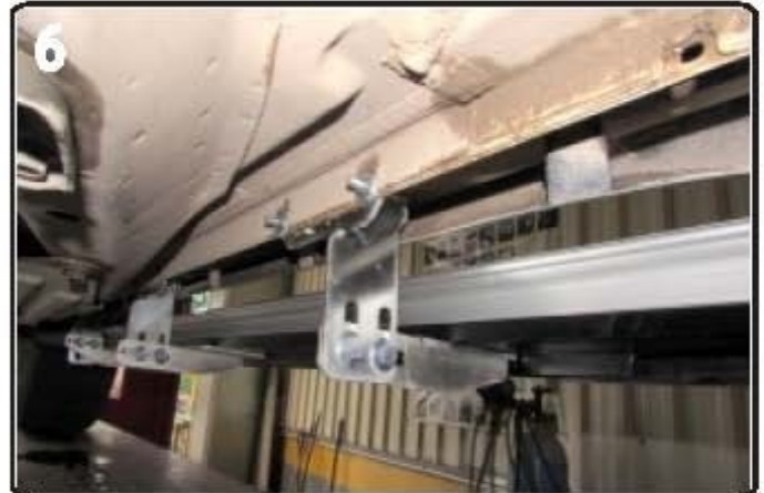
6) Properly installed brackets
