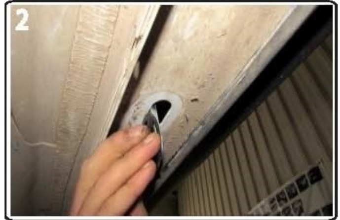
2) Remove rubber plug as shown above
