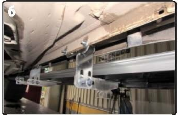
6) Properly installed brackets
