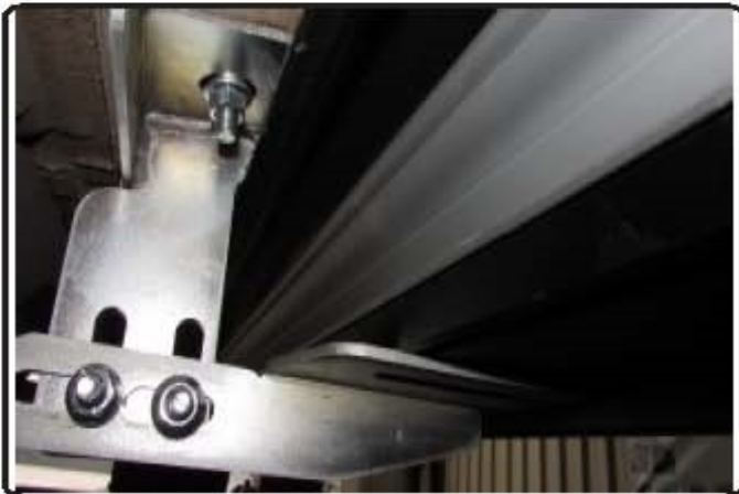
5) Attach lower portion with M10 hardware do not tighten yet
