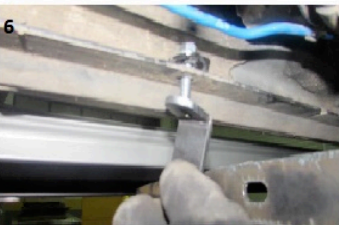
6) Install extra support bracket
