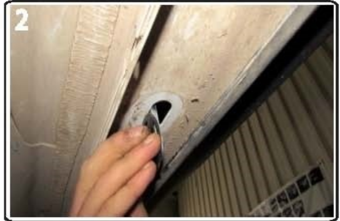
2) Remove rubber plug as shown above
