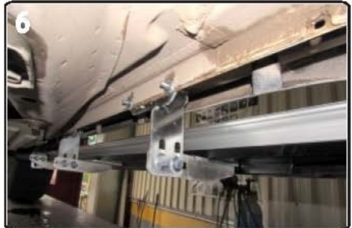
6) Properly installed brackets
