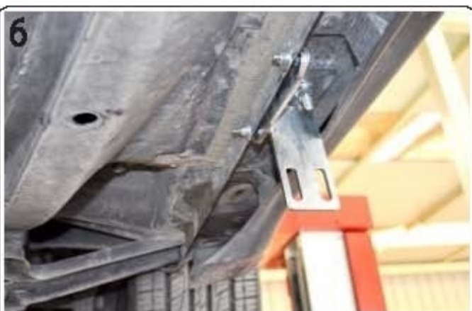
6) Bracket properly installed
