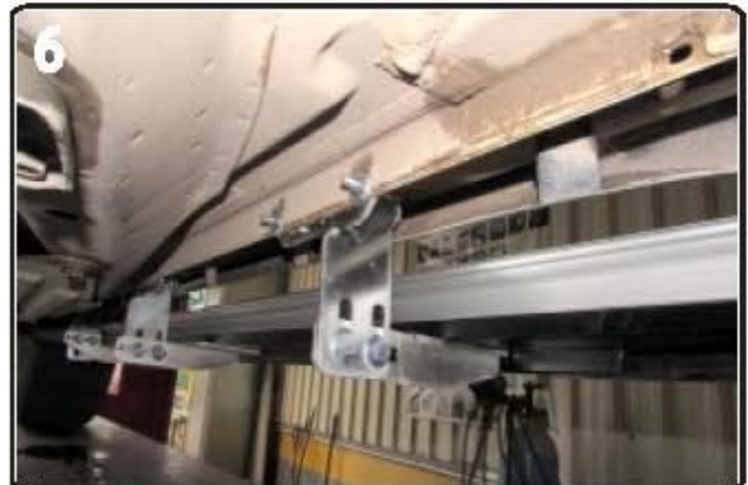
6) Properly installed brackets
