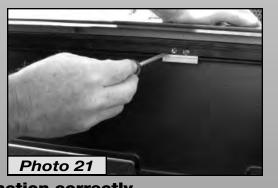
E. With the Tracks in the correct position, you may now tighten the Clamps (*Photo 21*). Do not use power or pneumatic screw gun.
