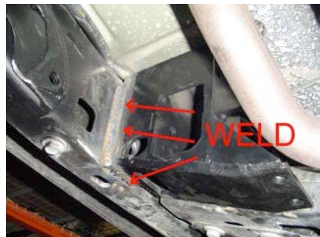
P.S. Bracket Welded in Place
