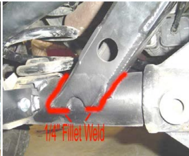
Welding the rear cradle
