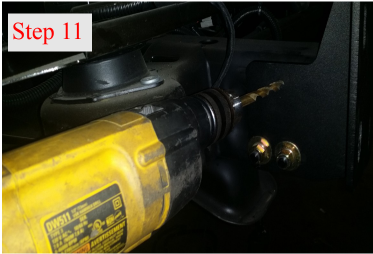
Step 11: Drill out pilot hole
