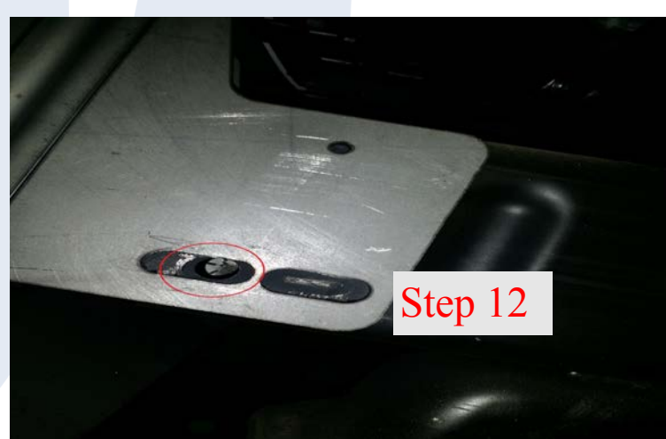
Step 12: Install bracket loosely with bolt tabs
