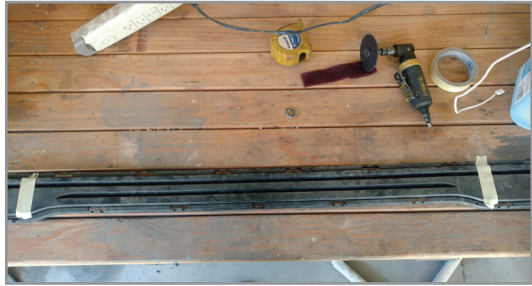
Vertical Cuts are Best Made from the Rear Face (30" Width Shown)
