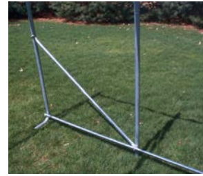
Structural wind brace on each corner
