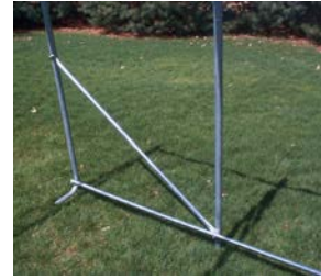
Structural wind brace on each side
