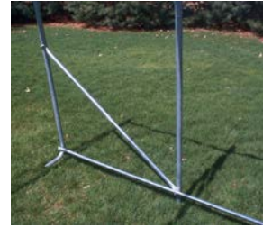
Structural wind brace on each corner
