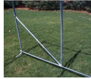
Structural wind brace on each side
