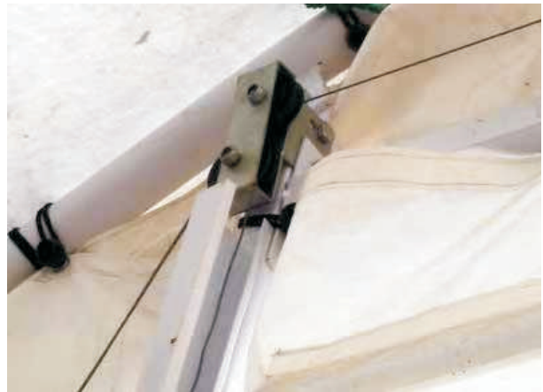
Double Pulley Nearest Winch Assembly
