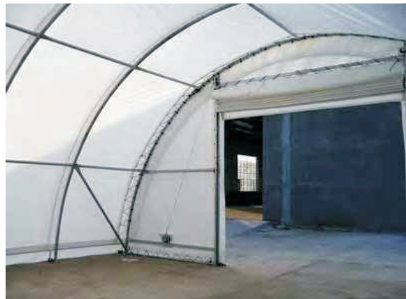
Main Roll Up Door in fully Open Position
