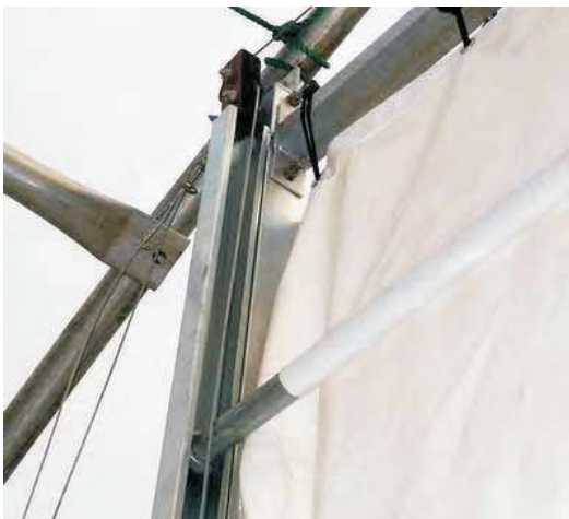
Door Tubes Inserted Into Door Track
