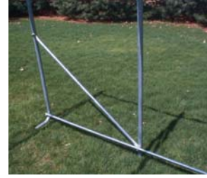
Structural wind brace on each side
