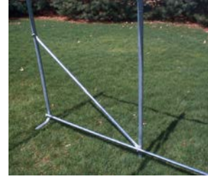
Structural wind brace on each side
