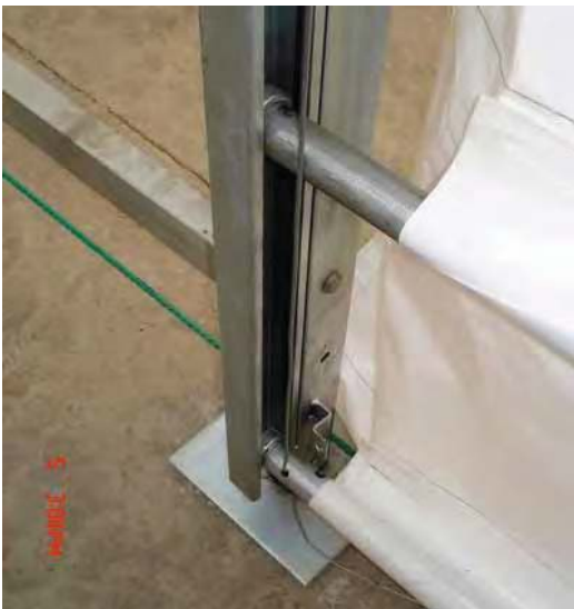
Door Tubes Inserted Into Door Track
