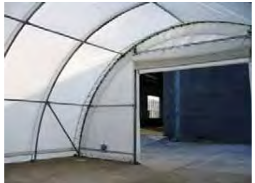
Main Roll Up Door in fully Open Position
