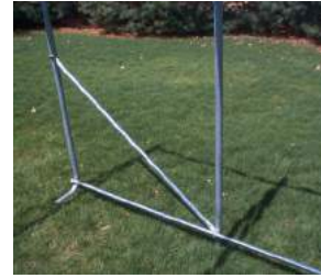
Structural wind brace on each corner
