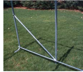
Structural wind brace on each corner
