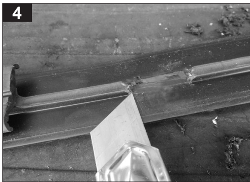
Trim excess rubber.
