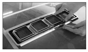
7.) Pull the front tab toward the opposite side of the vent as shown below. Apply firm pressure where the lining has been removed.
