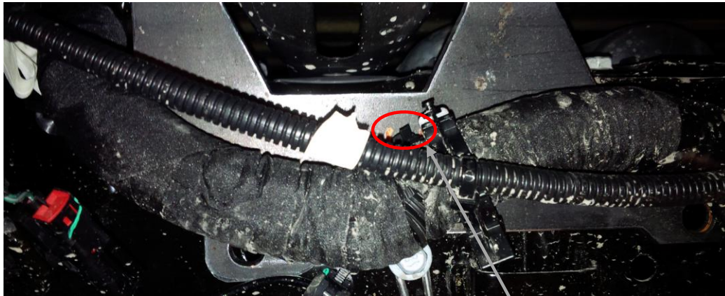
Driver's side - typical
