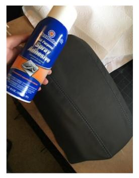
**6.** Using an automotive spray adhesive, spray top of foam armrest.
