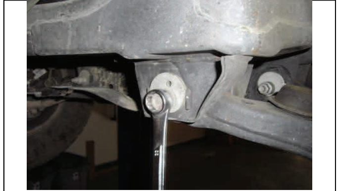
Reset and tighten lower control arm bolts
