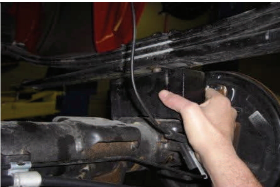
Lower axle more in order to install new lift block
