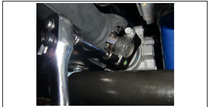
38. Re-attach front drive shaft using OEM bolts and straps.
