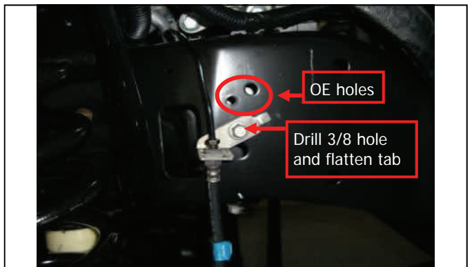
Shown, pass. side new 3/8 brake line hole location.
