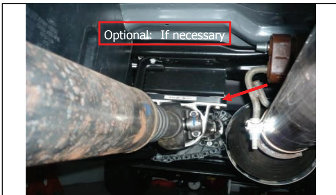
With vehicle on the ground install carrier bearing drop plate.
