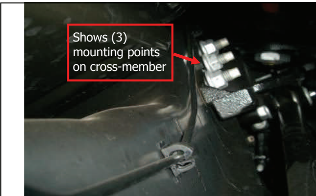
Install new bracket with factory hardware and torque to spec.
