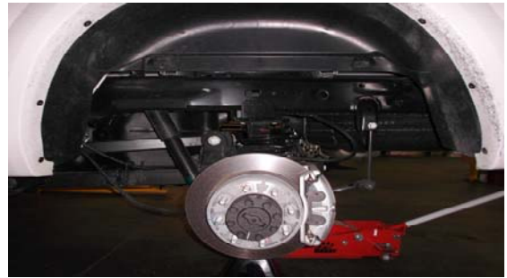
22. Lift the vehicle by the frame, support the axle, and remove the wheels.
