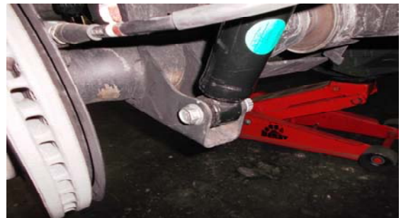
28. Jack the axle back up to weight the springs then install the shocks.
