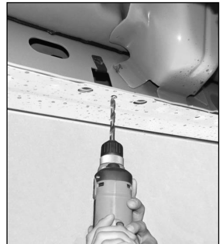
Figure 5. Optional: Mark to Drill for Center Bracket Mounting
