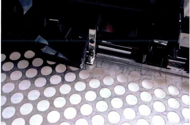
Step 9: Lay the Punch Grille in the surround making sure the grille is fully seated and all the gaps are consistent. Mark all the holes from the L bracket.
