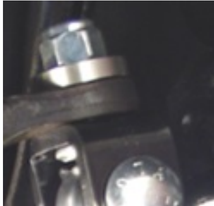
Billet Stainless Steel Washer Installed
