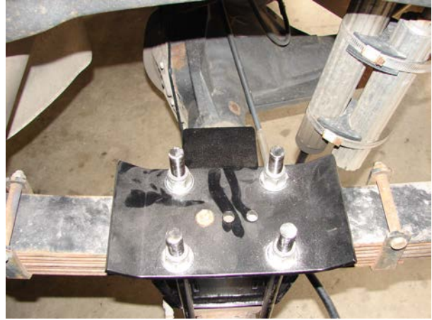
Top Plate and U Bolts Installed
