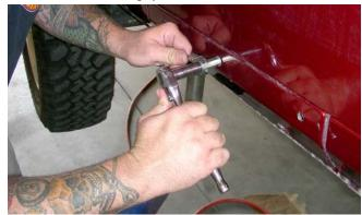
8. Once the nut-sert has seated correctly, loosen the bolt then remove it and the rest of the tool from the nut-sert. Install a new nut-sert onto the tool, oriented the same as the last, and set it aside until your next nut-sert installation.
