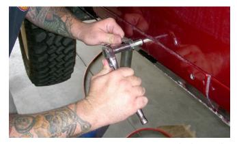
18. Once the nut-sert has seated correctly, loosen the bolt then remove it and the rest of the tool from the nut-sert. Install a new nut-sert onto the tool, oriented the same as the last, and set it aside until your next nut-sert installation.
