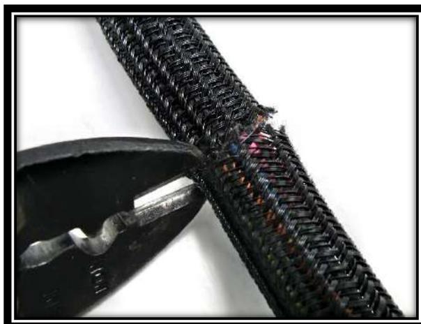
**Step 13:** Strip each of the **Switch Panel Wires**  $\frac{3}{16}$ ", and install a male pin terminal from the parts kit onto the end of each wire. See [page 4](#) for detailed instructions of how to properly crimp these terminals. We recommend [Painless #70900 Roll-Over Crimpers](#).
