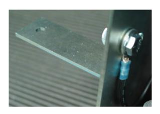
Loosely install the two metric capscrew's, lock washer's and flat washers supplied through the bracket, loosely install the capscrew removed from the ground terminal bar through the compressor support bracket. Tighten all the capscrew's evenly including the ½" nut and bolt under the compressor, make sure the compressor ground wire is tightened with the bolt.
