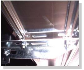
Place the board on the brackets with the bolts through the slots. Fasten with 1/4" nuts.
