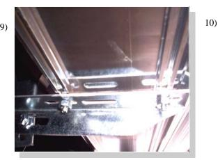
Place the board on the brackets with the bolts through the slots. Fasten with 1/4" nuts.
