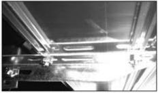
6.Place 1/4" bolts through bracket step support and secure board with 1/4" hex nuts.
