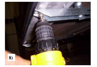
8) With board level and properly aligned, attach to the brackets with 3/4" long self drilling screws.
