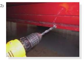
At each of the locations from step one, drill a 5/16" hole through the pinch weld, if no factory hole is present.
